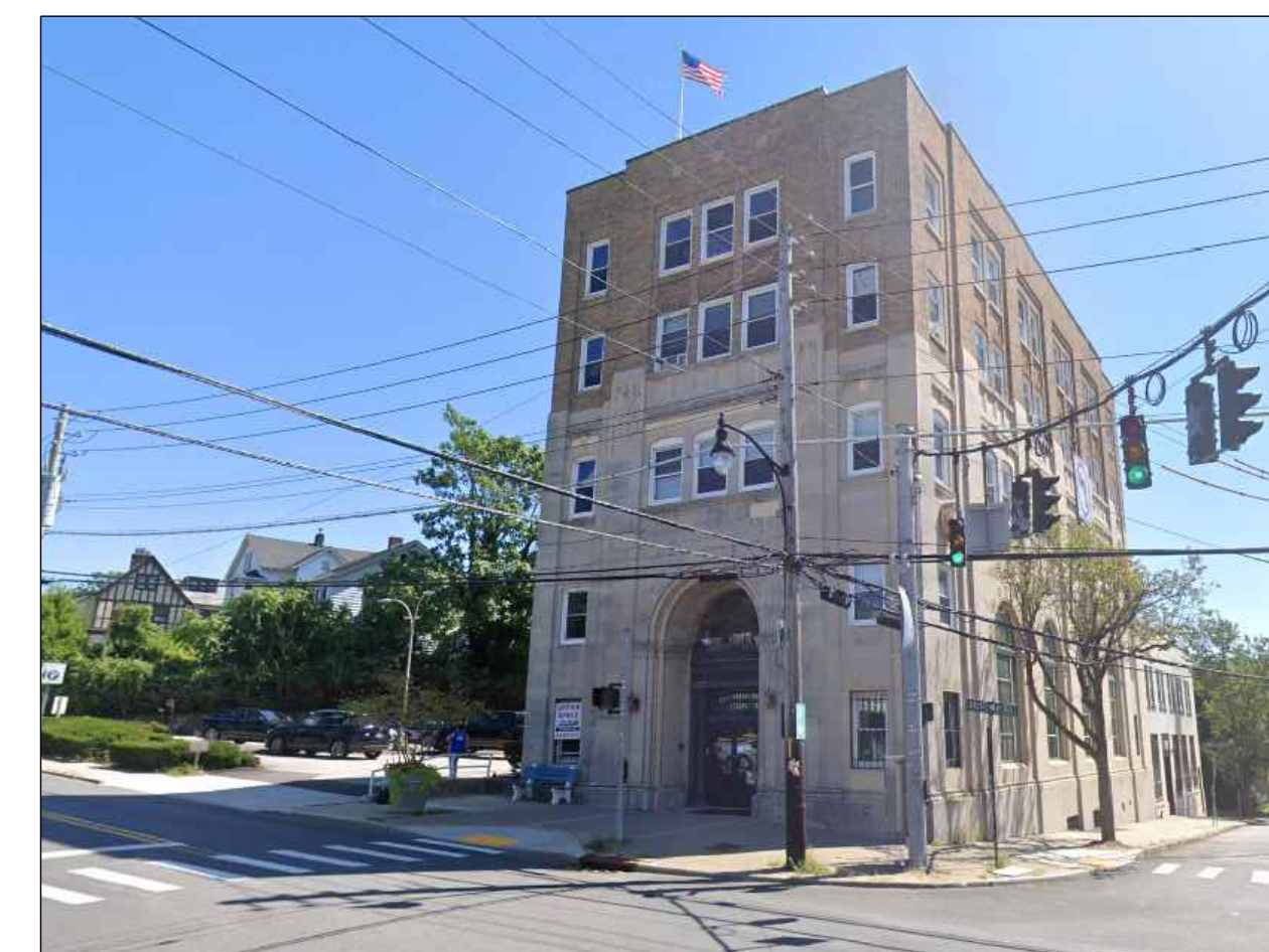
EXIST. BUILDING IN 2022 N.T.S.
