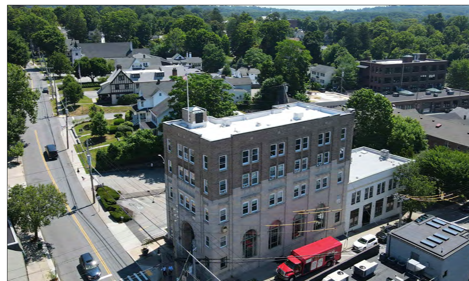
EXIST. BUILDING IN 2022 N.T.S.
