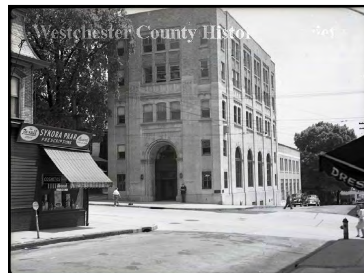
EXIST. BUILDING IN 1920 N.T.S.
