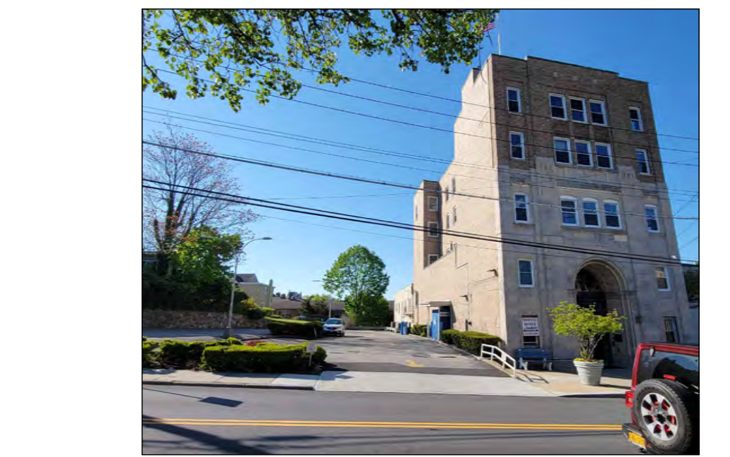
EXIST. BUILDING IN 2022 N.T.S.
