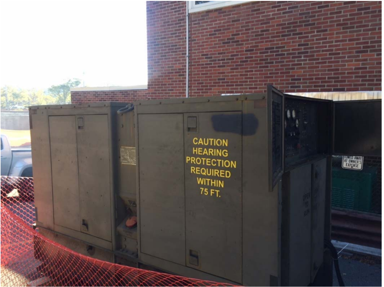
Existing 200kw Generator -which requires a manual start
